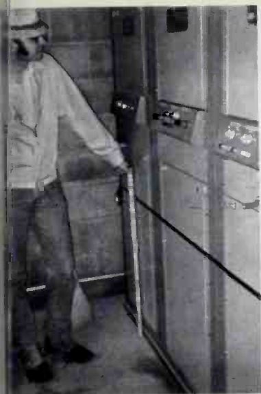
Fig. 1 Tape line on transmitter indicates the high water mark at the transmitter site.
