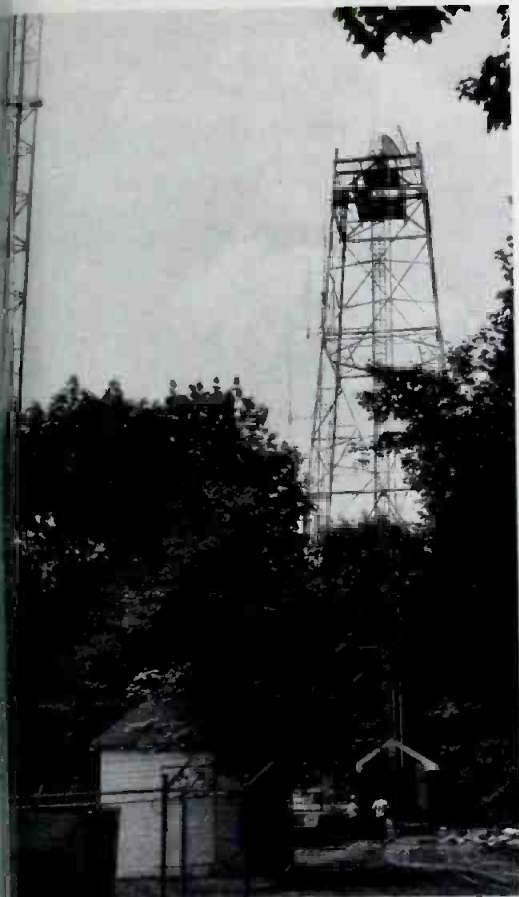
Fig. 3 Radar RF system at Avon, Conn. The range indicator had not been installed when this picture was taken.
