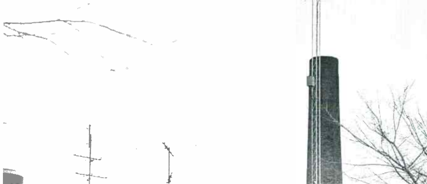
A typical receiving antenna installation shows tower and other components.
