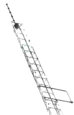
Omnidirectional transmitting antenna is side mounted with UHF unit on top.
