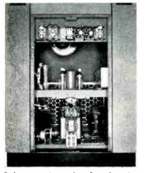
Relays are in a dust-free location. All components and circuit terminals are in convenient locations.
