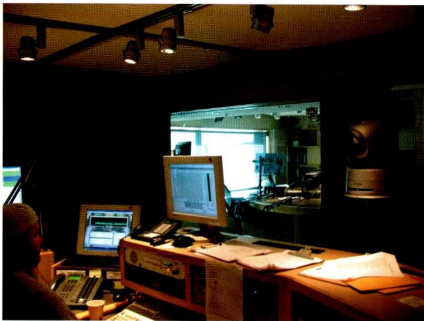
In Seattle, WA, KJR radio station made an agreement with Comcast SportsNet to broadcast TV content from its studio. Advanced Broadcast Solutions employed green practices when overhauling the space so it could be used for both radio and TV. The systems integrator installed Philips Kinetics LED lighting as well as robotic cameras.
