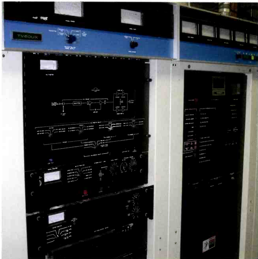
Shown here is a klystron analog transmitter used for KVTN Ch25 that was retired on Feb. 9, 2009. Not only is the transmitter old, but also the technology will not work on DTV economically. It is now being scrapped piece by piece, with some parts going to radio amateurs, while the rest are just metal scraps.
