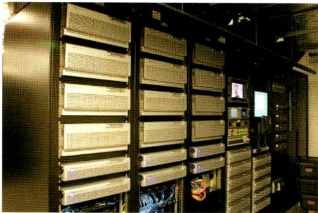
The Newseum in Washington, D.C., uses Grass Valley K2 media servers, which provide file-based, IT-centric storage.
