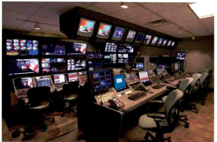
One of two HD control rooms, leftover from the MSNBC days, has been rejuvenated with a Sony MVS-8000G HD video switcher, Miranda Kaleido-X multiviewer running on 13 Sony 42in flat-panel displays in each, and a Calrec Omega digital audio console. Both rooms will be used simultaneously during the baseball season.
