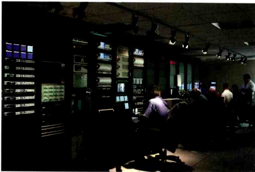
The central machine room houses 18 racks and space for personnel to work for studio productions, with ample room for expansion.
