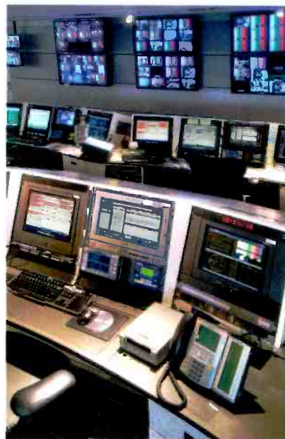
Master control operators share various duties across eight stations, including ingest and playout and feed monitoring.
