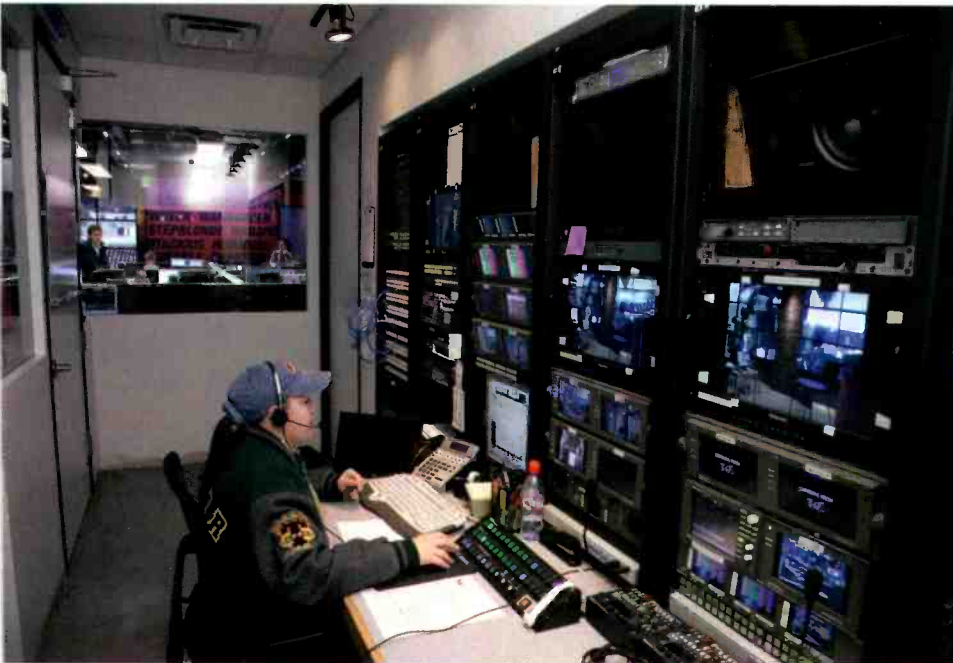
Traffic coordinator Kerry Moynahan works in the master control suite, where the recording of all incoming feeds and automated playout of TMZ programming occurs. The suite also handles production control and transmission operations via an NVISION 64 x 64 router.
