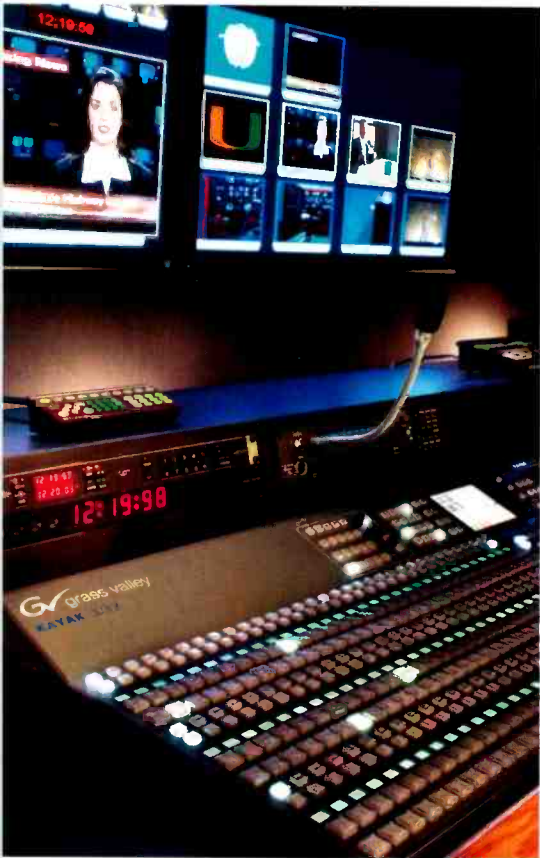
Three 50in Panasonic high-definition plasma panels are driven by Miranda Kaleido multi-image systems, enabling signal input from any source and unlimited custom configurations. They also show audio levels and on-air tally. The console is a Grass Valley Kayak production switcher in a 2.5 M/E configuration.
