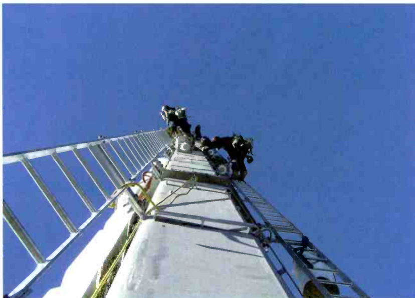
Radio Frequency Systems' PHP30C directional antenna at Mt. Wilson in Los Angeles uses a five-sided steel structure with antenna panels on three faces.
