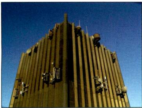
One Boston Place, the most popular ENG site in downtown Boston, is scheduled for some major work during the 2GHz relocation. Photo courtesy of WCVB.
