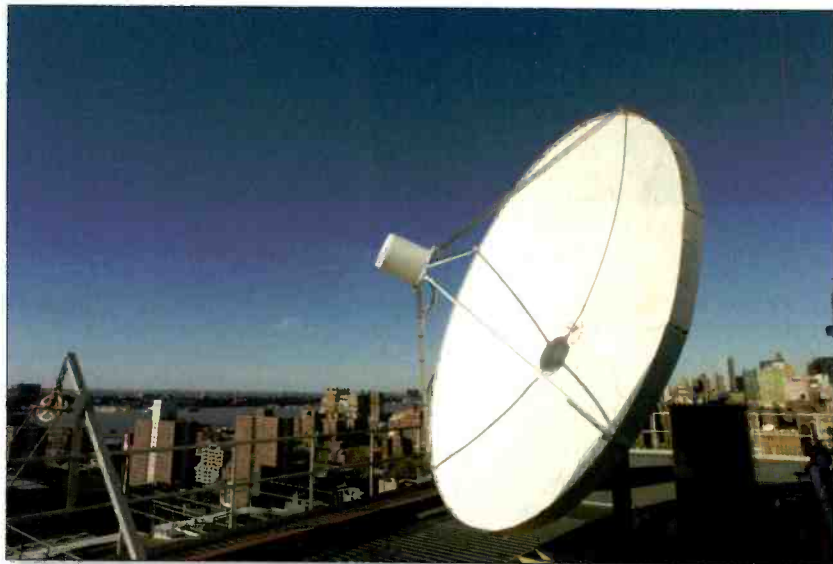
Two 3.8m TVRO antennas monitor Lifetime's satellite downlinks.
