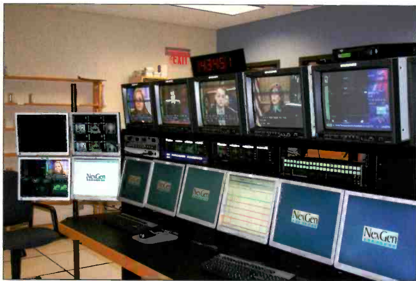
This TOC provides operations for KOKI-TV and KFTO-TV in Tulsa, OK, KVOS-TV in Bellingham, WA, and KFTY-TV in Santa Rosa, CA. NexGen software is stored on the video players, as well as all control and ingest stations.
