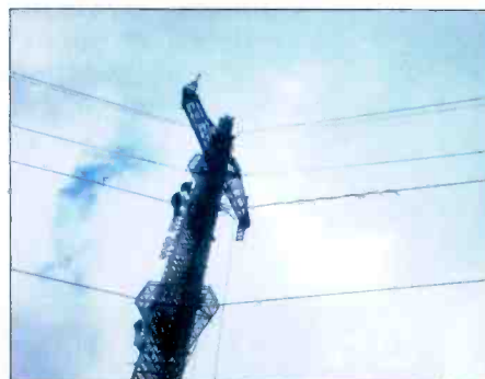
After a major storm, an intact tower can help to make a broadcast station available for emergency communications.
