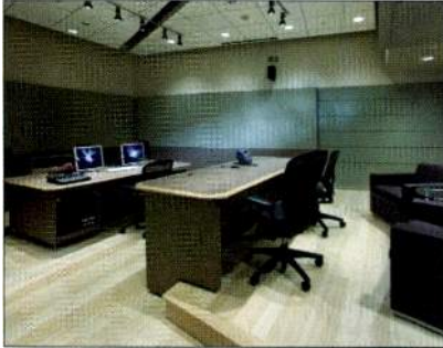
The bamboo flooring in the audio suites and video-audio control rooms sits atop a dual floating concrete slab foundation. This, along with the sound absorbing material on the walls, makes for an ultra-quiet working environment.
