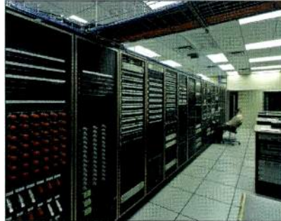
The central machine room is the main hub from which all processes take place. Noise is kept to a minimum within the surrounding edit suites because routing, patching and tape playback occur in this area.
