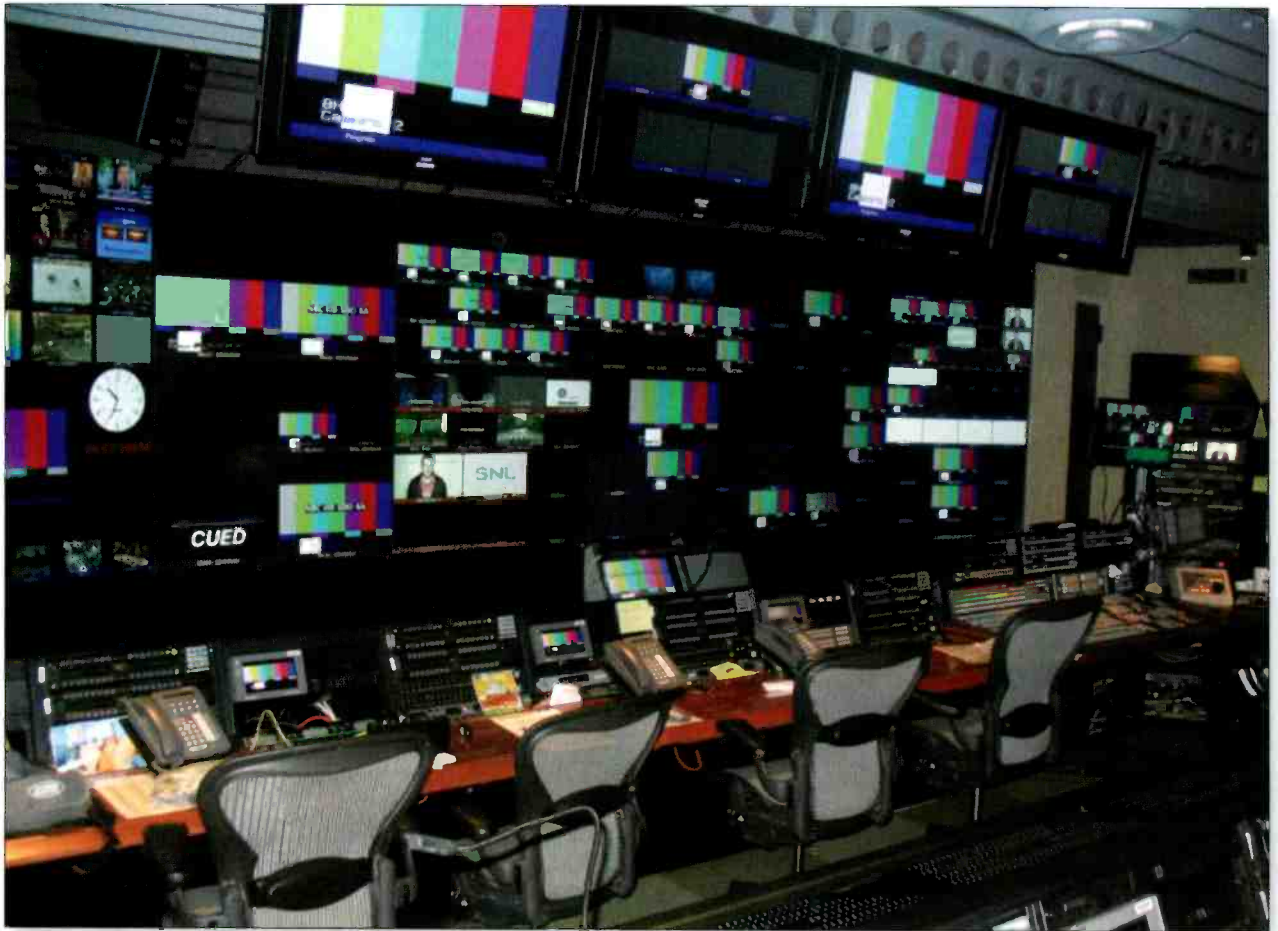
The new NBC Universal Studio 8H production control room in New York City's Fockefeller Center is equipped with the latest HD video and digital audio technology. These systems get their timing reference from redundant master signal pulse generators locked to GPS receivers that are fed from dual antennas atop NBC Headquarters. Photo by Jim Starzynski.
