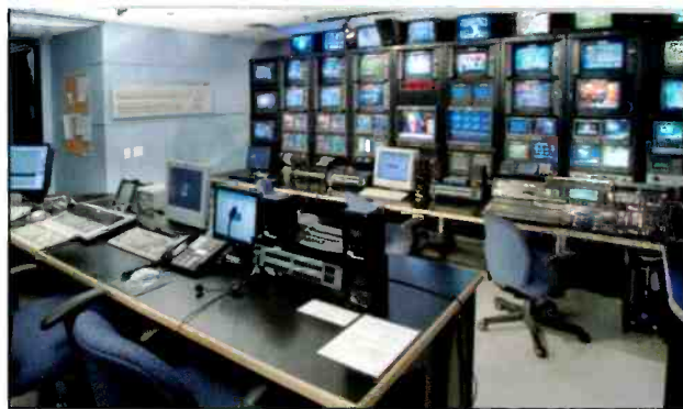
The production control room is supported by a 24-channel Allen-Heath audio console, a Ross Synergy 3 production switcher and a two-channel Abekas DVE. A Chyron HyperX CG is currently being installed.
