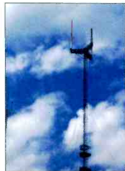
Richland Towers' dual-purpose antennas on the Richland Atlanta broadcast tower stand 120 feet above the tower. The stack on the left shows these two broadband antenna systems, both carrying DTV and NTSC signals.
