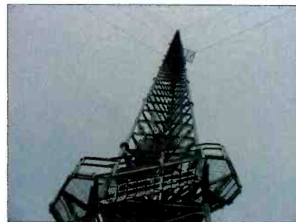
KMOS's new 1925-foot tower in Tipton holds a digital slotted-line antenna at the very top and an analog three-faced panel antenna at 1860 feet.
