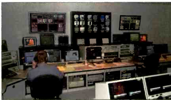
The transmission room at WLS-TV in Chicago functions as the news ingest and feed room for all microwave and satellite links.
