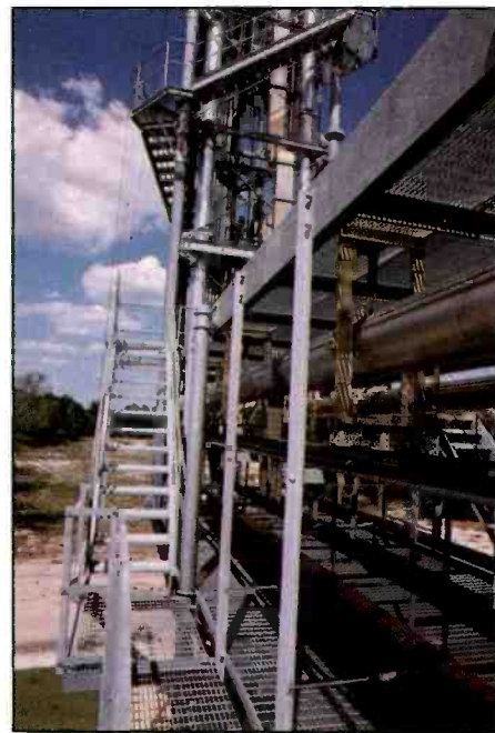
The Dielectric truncated waveguide allows the transition from coaxial cable or rectangular waveguide to be made in the transmitter room.
