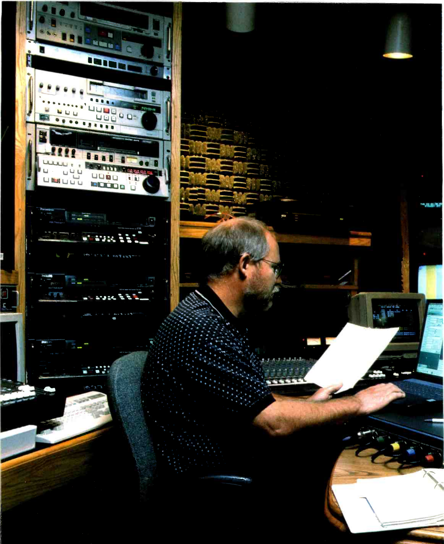
Pat Shearer, chief engineer at KWBP in Beaverton, OR, monitors the quality of the station's audio signals from the studio control room.
