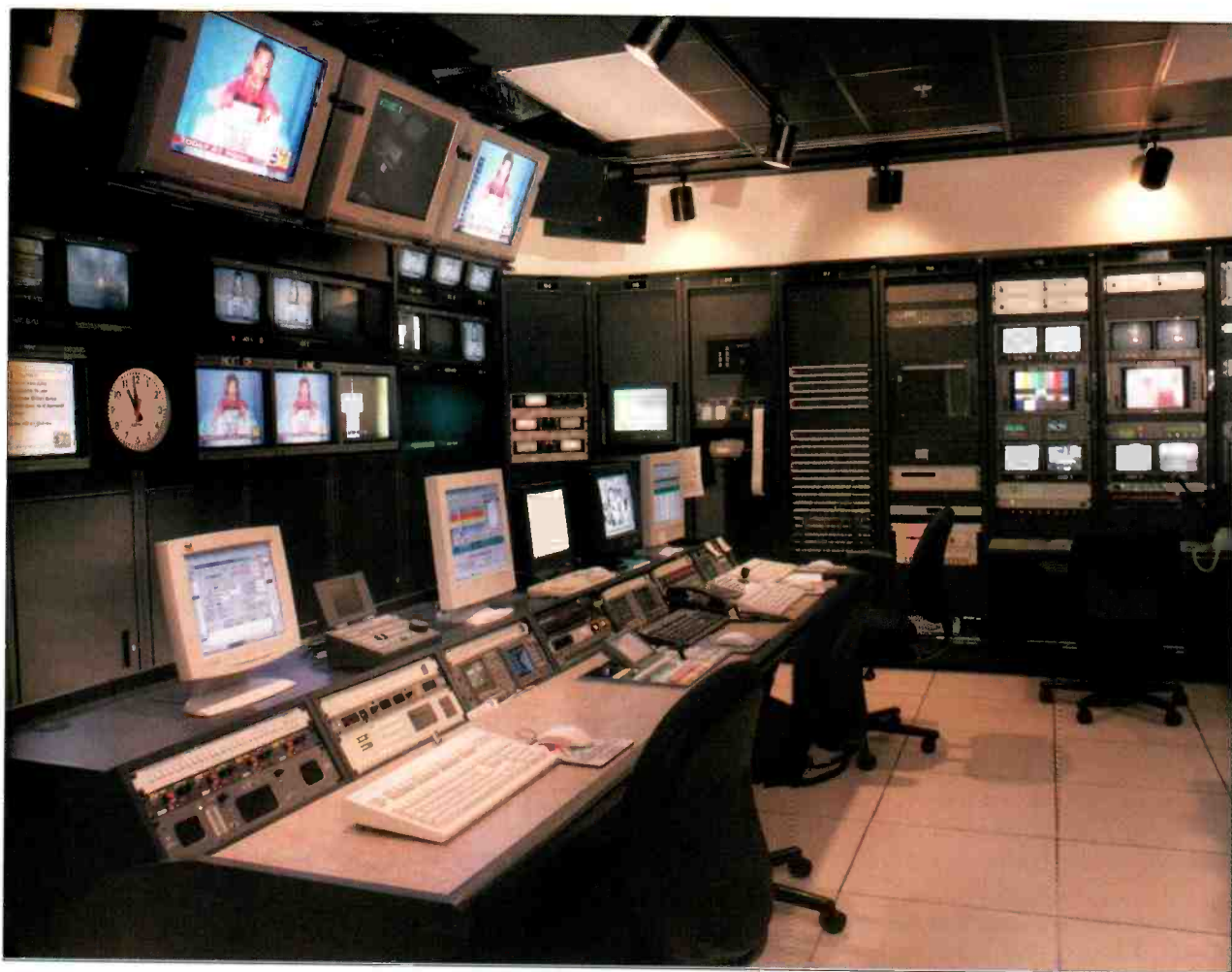
The master control room at WWSB Channel 40 utilizes Sundance Digital's Intellisat to control the Omneon networked content server system for satellite ingest. Also displayed are the Sundance Fastbreak on-air and prep stations.
