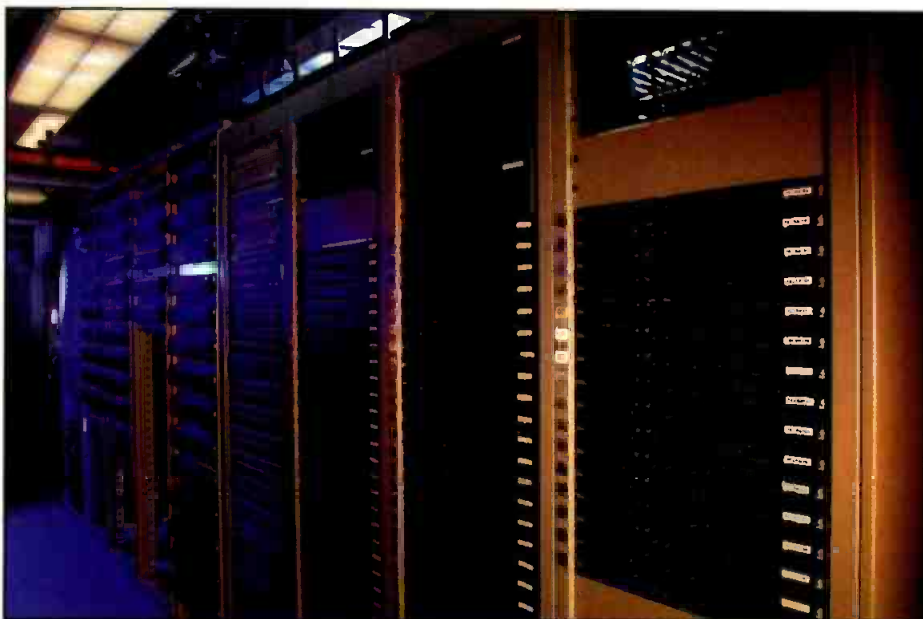
Racks of Symetrix 422 and 221 auto-levelers and other terminal equipment. The Symetrix units feature adjustable auto-leveling and automatic gain control.
