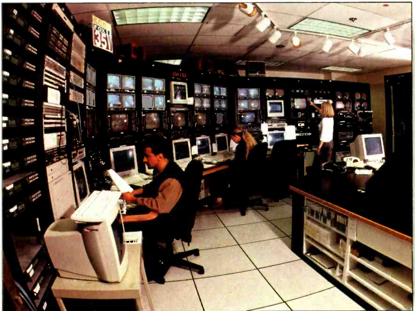
KCBA utilizes Sundance Digital automation, DPS A/D converters and a SeaChange Broadcast MediaCluster for short-form programming.
