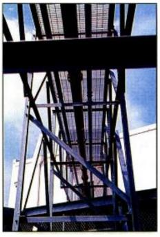
In an effective rigid line installation, the minimum length of a horizontal run of rigid transmission line (shown above) and the minimum distance to the lowest vertical spring hanger must be carefully calculated to compensate for expansion and contraction in the vertical and horizontal runs.
