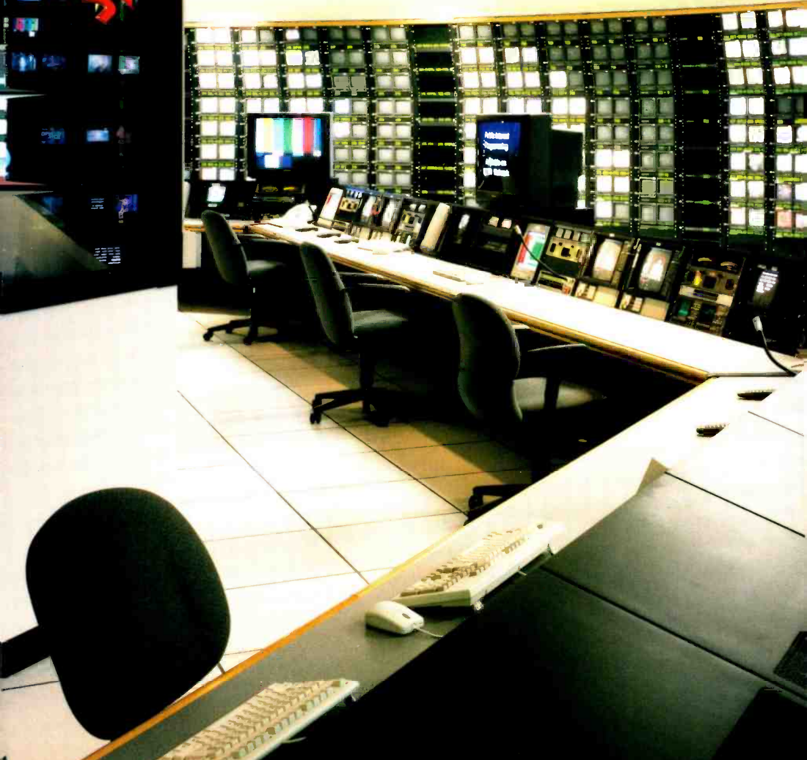
EchoStar's Satellite Uplink Center in Cheyenne, WY, monitors over 500 digital direct broadcast satellite channels. The Network Operations Center is equipped with 1020 receivers and 1020 JVC monitors. Photos courtesy of IMMAD ECVS.
