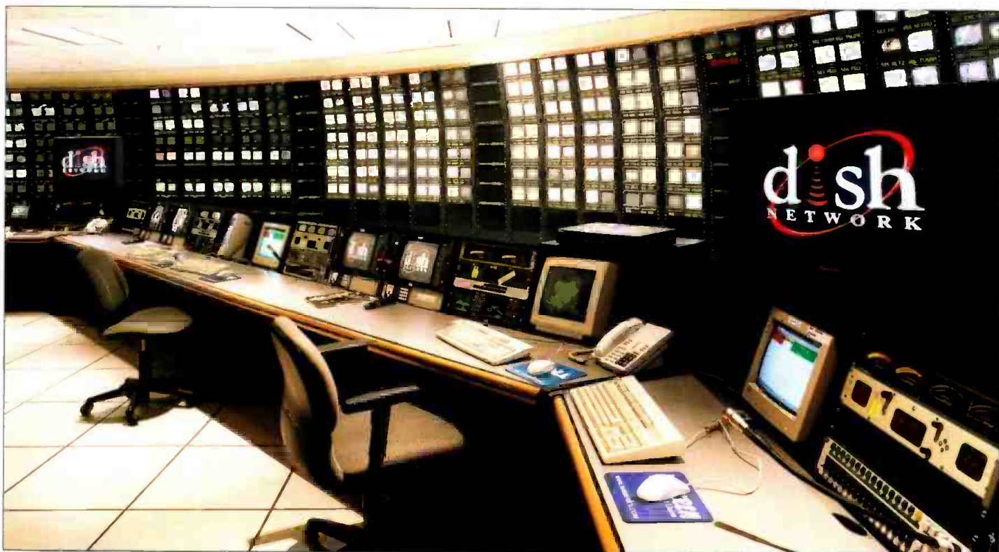
Operators assess quality control from confidence receivers in the NOC. Signals to the receivers are routed by a Grass Valley Group digital 1024x128 monitoring router, through GVG A/D converters and to Leitch analog video and audio DAs.
