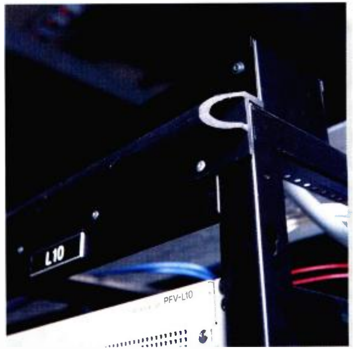
Close up of the rubber shock absorber on the tops of the racks. These are designed to soften the impact if the rack tops contact the sides of the container.
