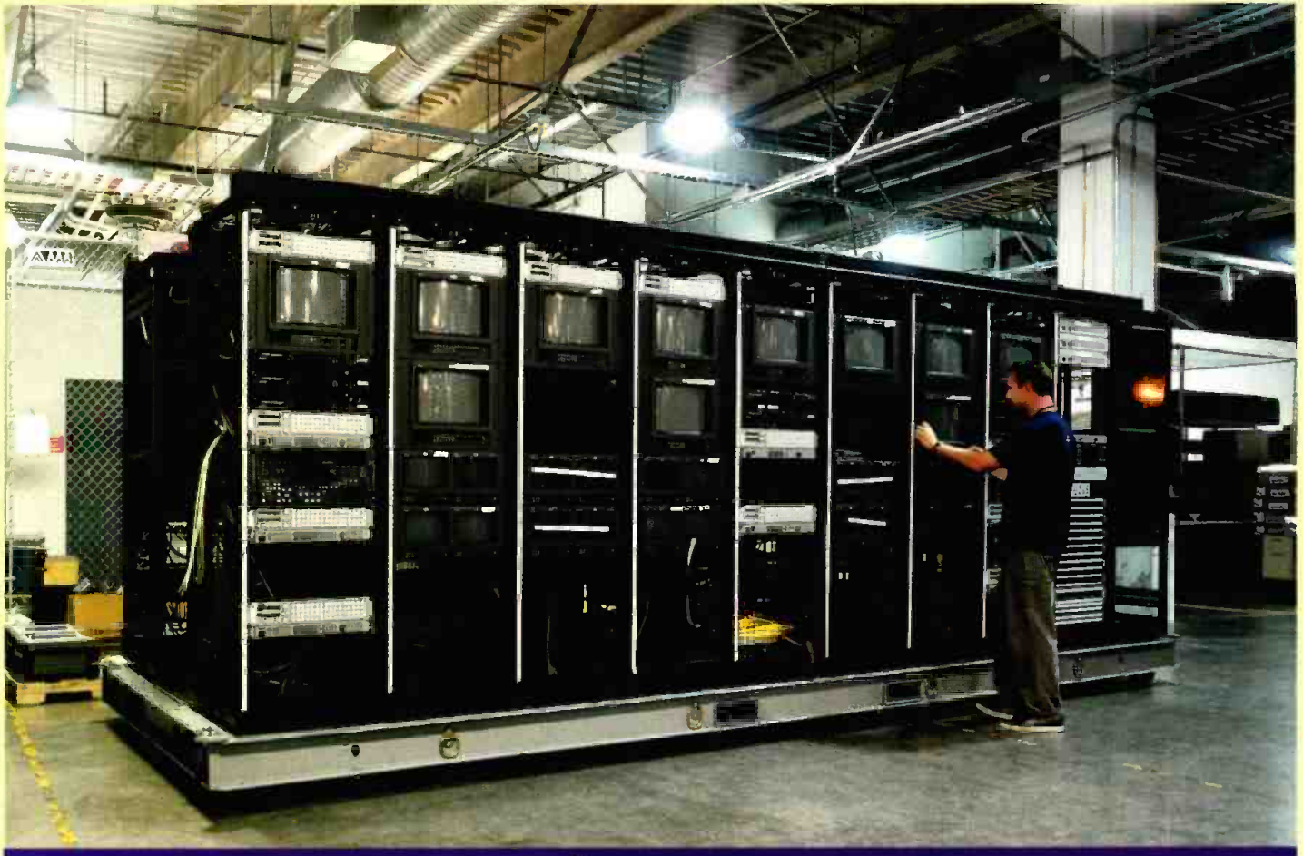
One of the nearly completed RIBs undergoing some last minute touch-up before final inspection and preparation for shipment. Photos courtesy Concept: Benson & Rice.
