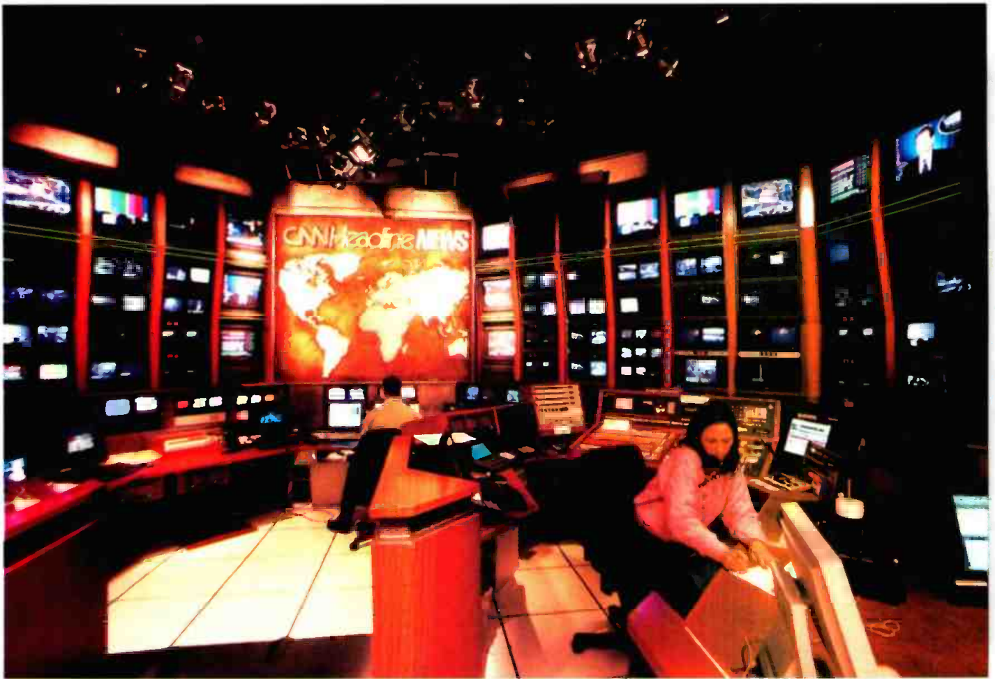
Control room for CNN Headline News. The main technical operating position, shown on the right, uses a GVG 4000 production switcher
