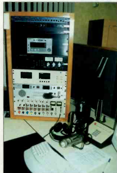
The news workstations are compact but still flexible. Notice the auxiliary audio jacks on the clock/timer panel.
