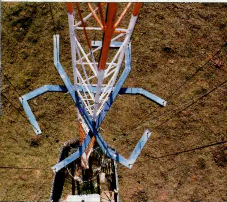
A view from above. The blue arms are insulating spacers.
