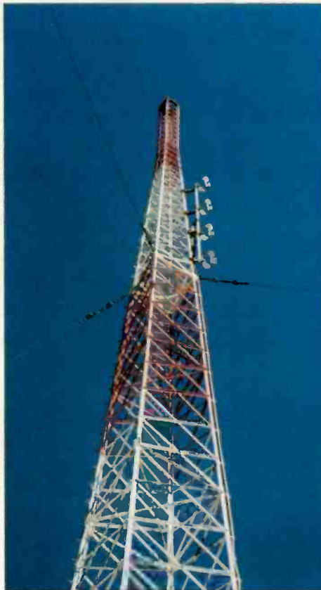
Metal guy wires should be kept clear of FM antennas so as to not interfere with their radiation.
