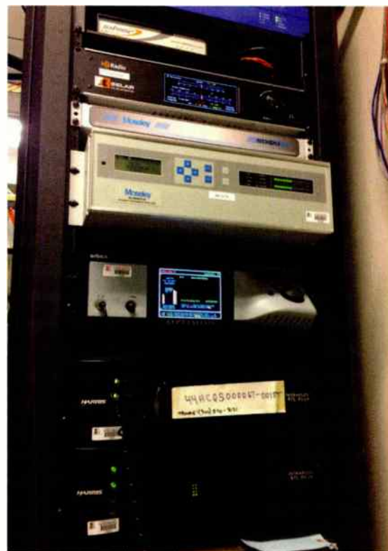
Top half of program distribution rack at KCSN, with Belar FMHD-1 monitor, Moseley 950 link to out-of-market translators, Orban Optimod 8700i and the former primary STL T1 frames.
