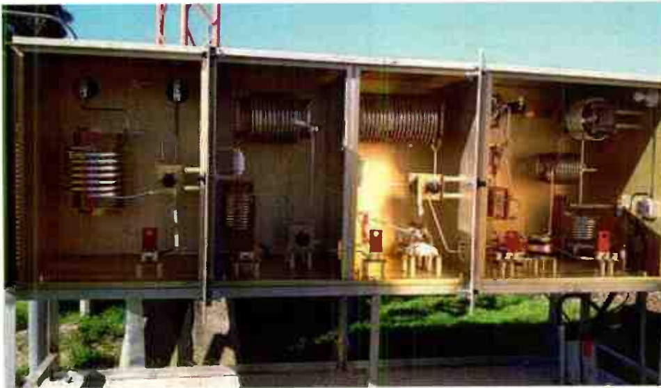
An ATU and filter combination manufactured by Phasetek.
