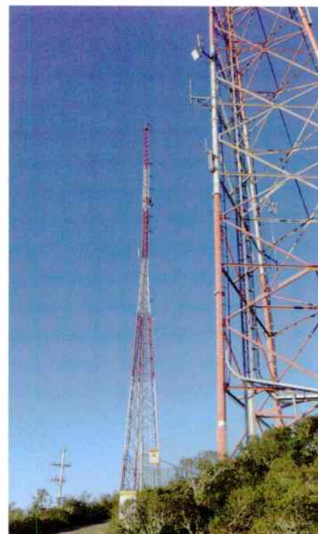
Overall view of the tower supporting the KQED(FM) antenna
