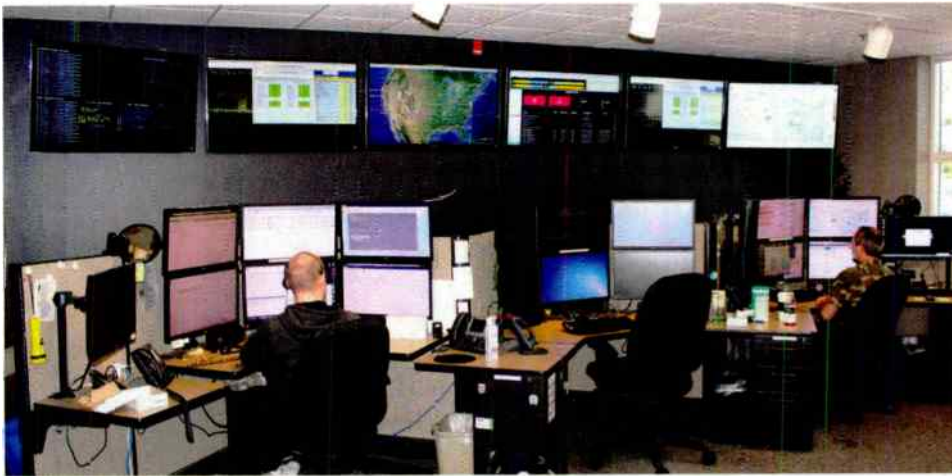
The EMF Network operations center is located in Rocklin, Calif.
