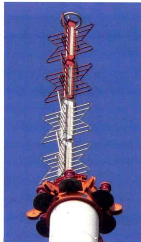
Many batwings are still in place, just waiting to be re-energized.
