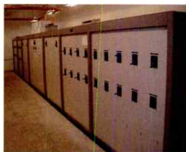
CUSTOM PHASOR INSTALLATION
