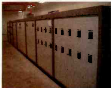
CUSTOM PHASOR INSTALLATION
