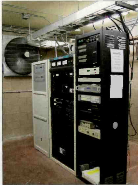
Everything installed and back on the air
