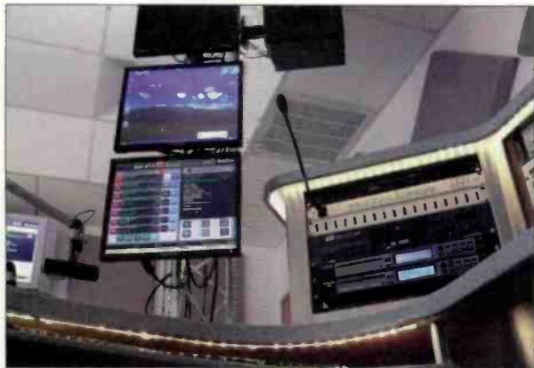
A channel was made under the counter lips to accommodate the LED rope lighting.
