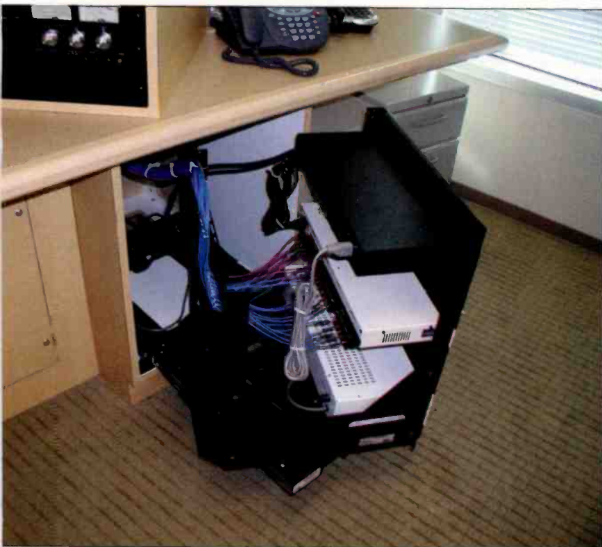
The Middle Atlantic slide-cut rack allows easy access to a tight space.
