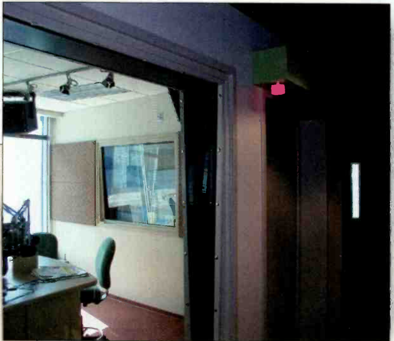
The on-air lights are mounted over the doors. The color contrast and flashing light increase their visibility.
