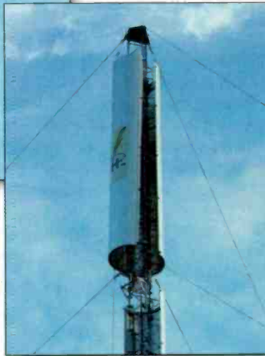
The EH antenna as it was being assembled.
