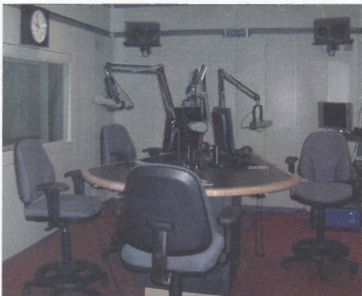
Studio B's pie wedge table arrangement makes excellent use of space for talk programs while offering flexibility and control. The studio can be operated from Studio 2, through the left window and Studio 3, through an identical window on the right.
