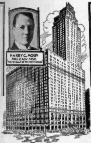
The New Morrison, when completed, will be the world's largest and tallest hotel—46 stories high with 3,450 rooms.
