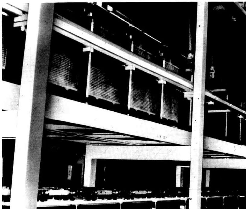
Fig. 5—Soft-site battery stand modified for service in earthquake area.
