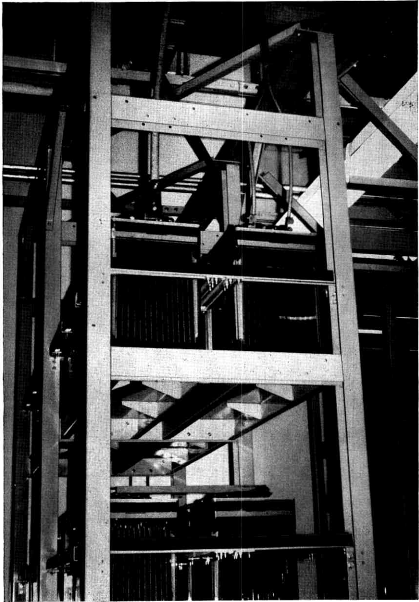
Fig. 4—Battery rack designed for earthquake areas.
