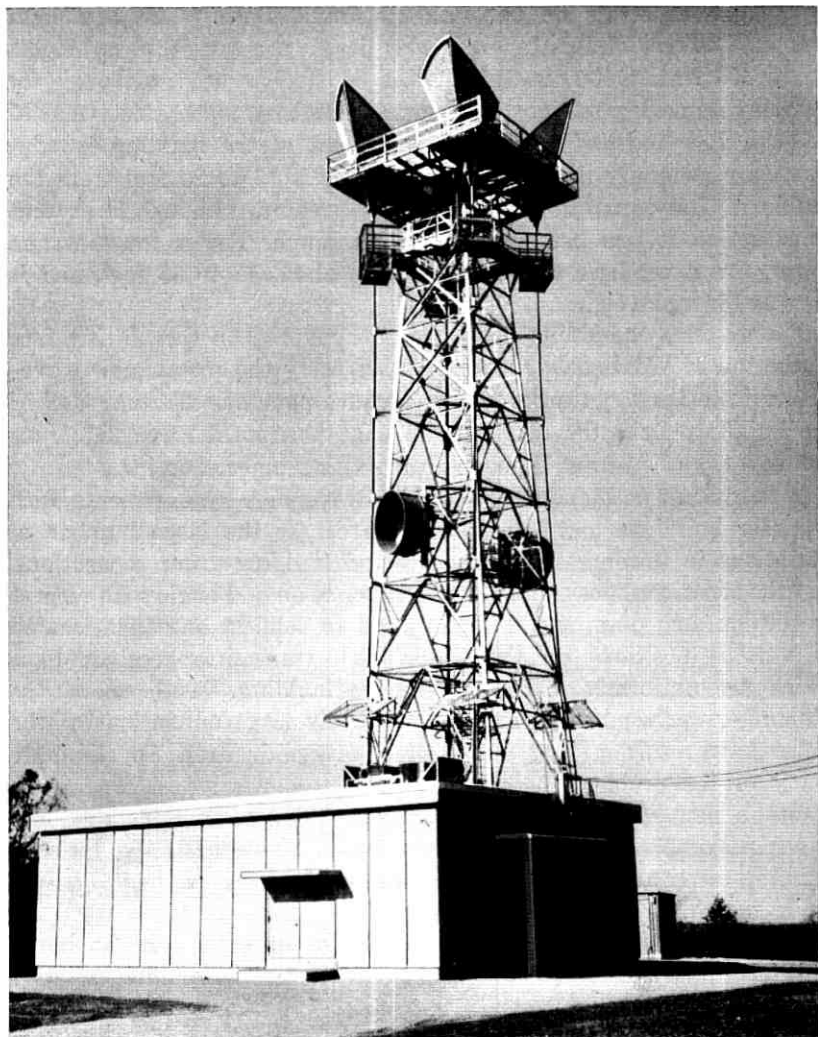
Fig. 9—This installation at Dumas, Mississippi, is typical of current TD-3 repeater stations.
