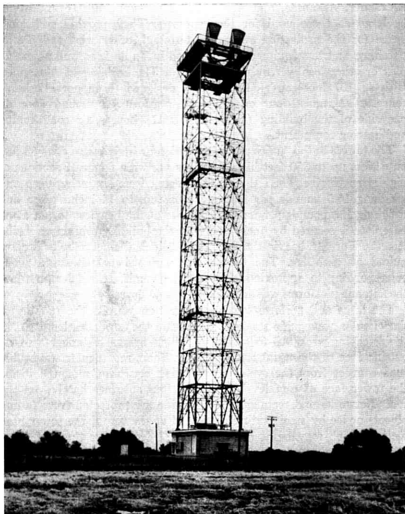
Fig. 10—The repeater station at Stuttgart, Arkansas, on the initial TD-3 route, uses a "unitized" building-tower arrangement.
