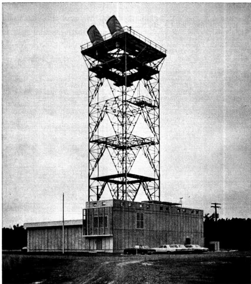
Fig. 11 — The main station at Alexander, Arkansas, on the initial TD-3 route.
