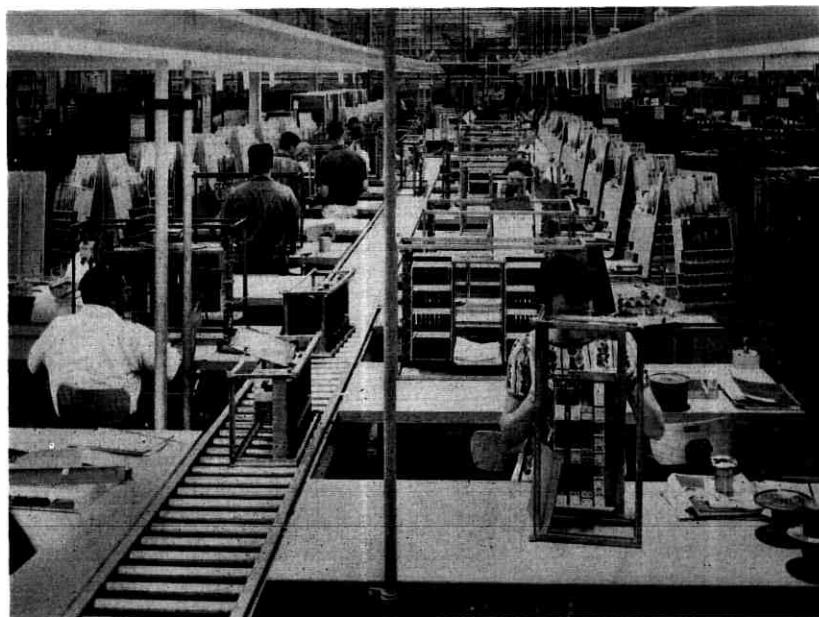
Fig. 41 — Western Electric Company manufacturing operations: unit surface wiring.
