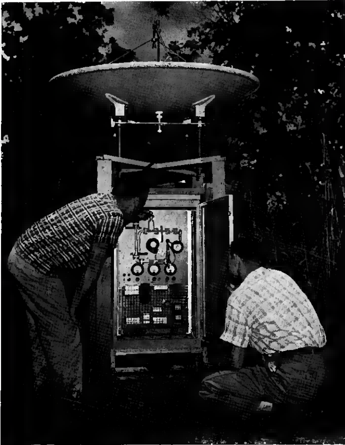
Fig. 16 — 11-kmc transmitter, power supply and antenna, Mount Vernon, Alabama.
