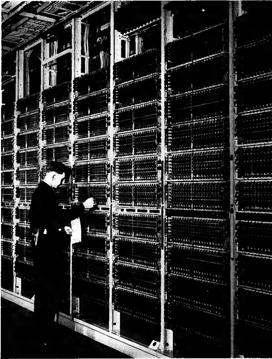
Fig. 18 — Part of a crossbar switching system.
