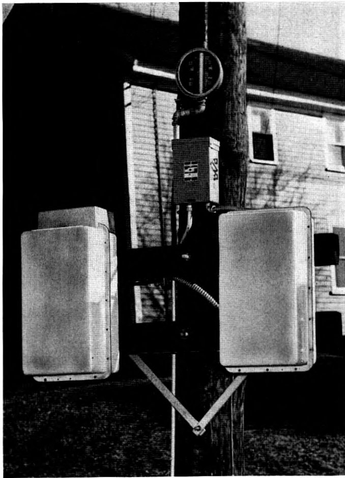
Fig. 20 — Example of remote mounting of P1 terminal and ac power supply.
