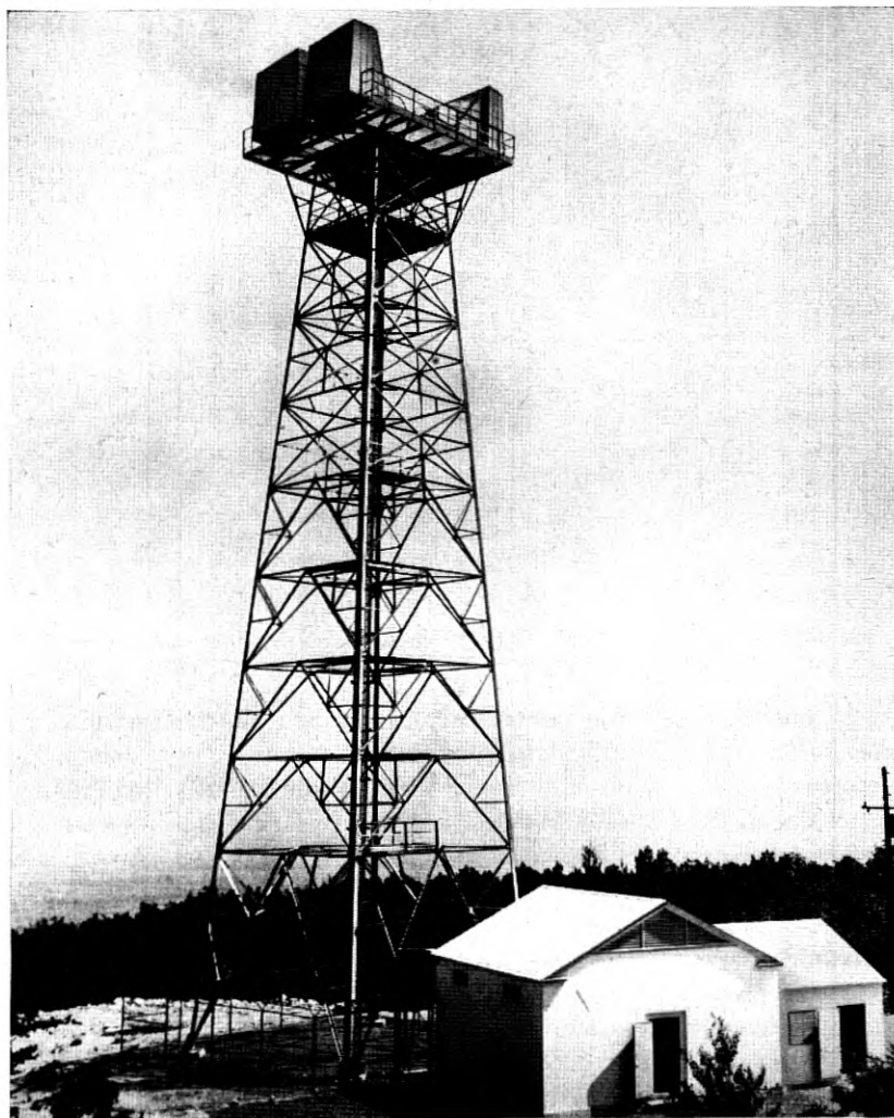
FIG. 10—Microwave radio relay tower at Cotocin Mountain, Maryland, on a New York-Washington radio route. There are 300 message circuits in service with more planned.
