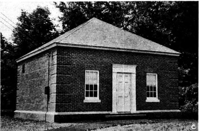
Fig. 8—Auxiliary repeater station buildings: A, without trim; B, with limestone trim; C, with limestone trim and artificial windows.
