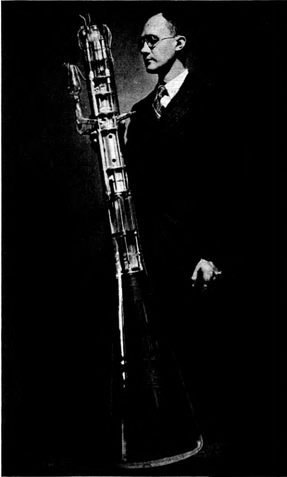
Fig. 10—Photograph of one of the special cathode ray receiving tubes.
