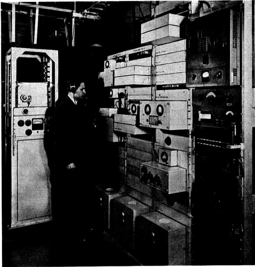
Fig. 13—Photograph of the transmitting carrier television terminal with associated sound apparatus.
