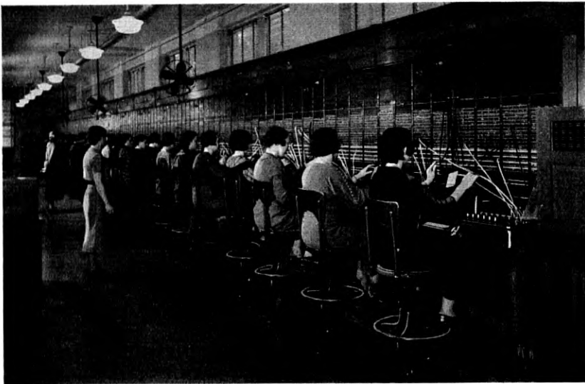
Fig. 1—No. 1 Teletypewriter Switchboard at New York, N. Y.
