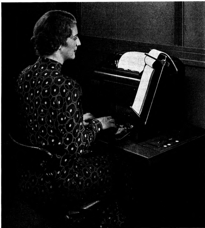
Fig. 9—Typical teletypewriter subscriber equipment for attended service.
