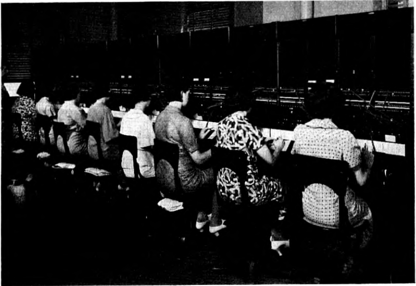
Fig. 6—No. 3A Teletypewriter Switchboard at Pittsburgh, Pa.
